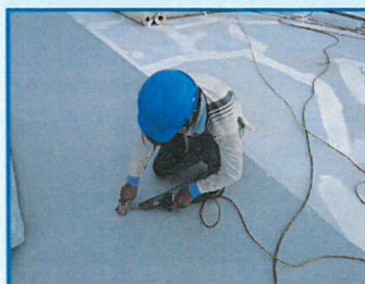
PVC防水膜鋁槍焊接
