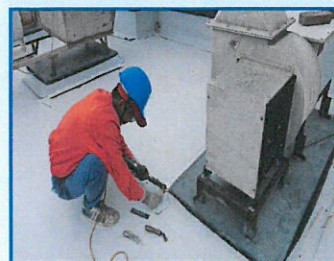
墩座PVC防水膜收邊
